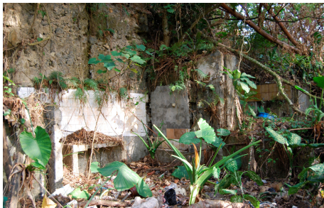
Tiles from the interior of a knocked down house.
