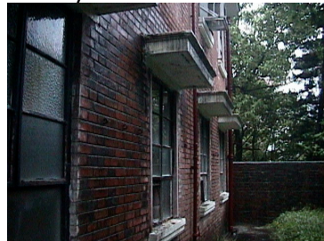
Figure 2 Side of Building
